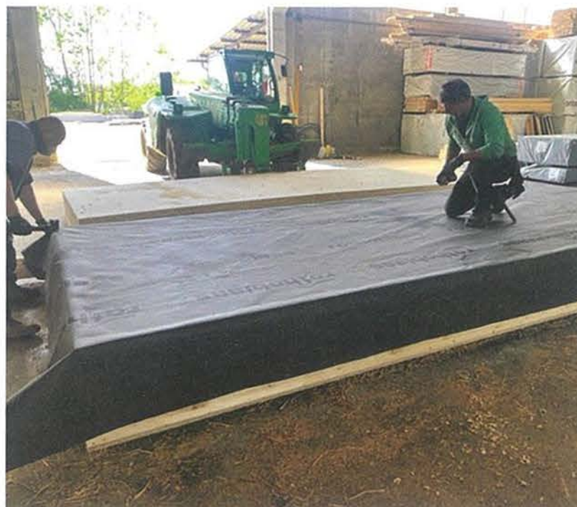
Pannelli preassemblati completi di guaina Preassembled panels complete with sheath
